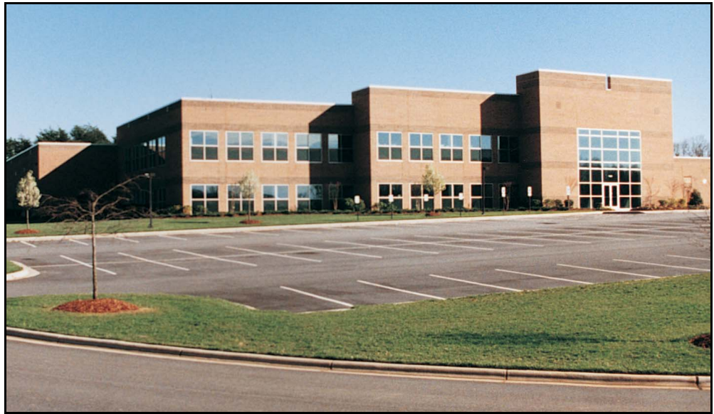
Dudley Products includes office, laboratory and manufacturing space. The solution to the diversity in loads was 13 heating and cooling air-to-air heat pump zones. Six zones were created for the offices and seven zones for the manufacturing plant.
